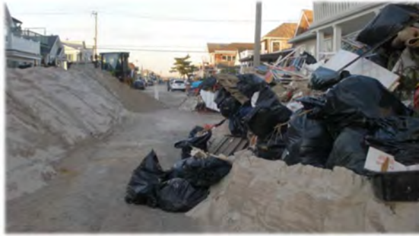
Pre-Segregation Debris Piles
