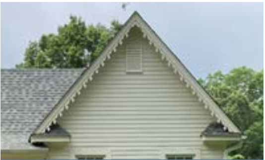
New construction in 2019 at 1224 Johnson Avenue
